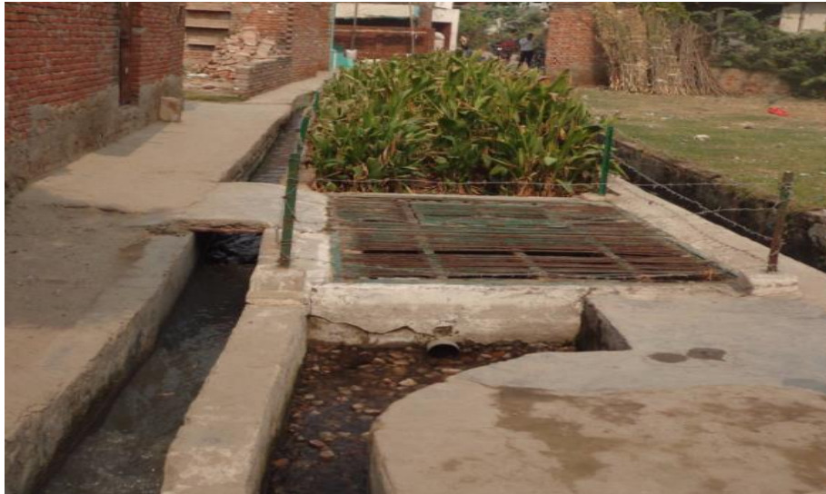
Figure 3.18 (DEWATS) was built by CURE over the Kuchpura drain.
