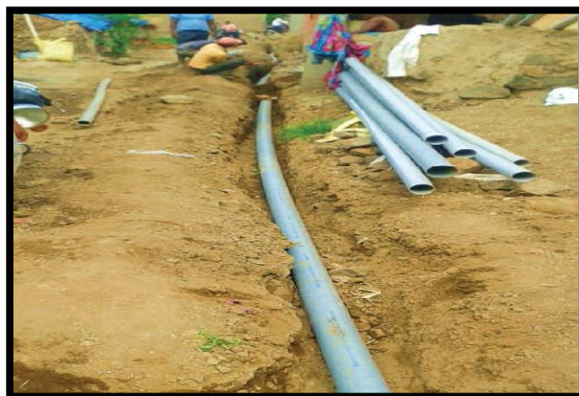
Figure 3.20 Laying down of Bore Lines
