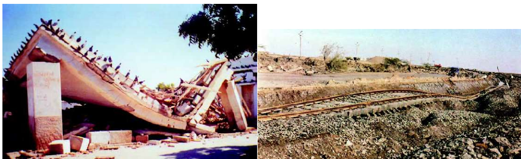
Fig 2.3: Damaged Bus stand near to Epicenter of Earthquake Damaged Railway line (Source: Pramod K. Mishra., 2012)
