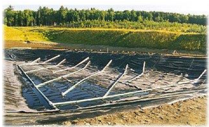
Fig 3.9 Preparing the base of the reed bed
