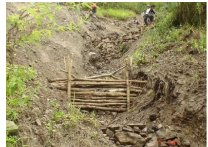
Fig 4.3 Gully plugging with bamboo
