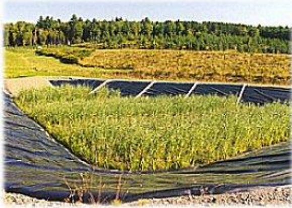
Fig 3.8 Sludge Treatment using Reed bed
