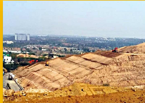
Fig 2.19 Step 3- Capping, geotextile awaited
