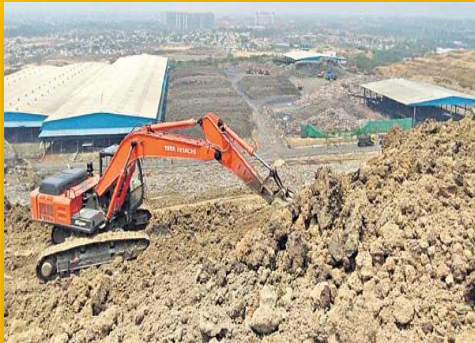
Fig 2.18 Step 2- Terracing
