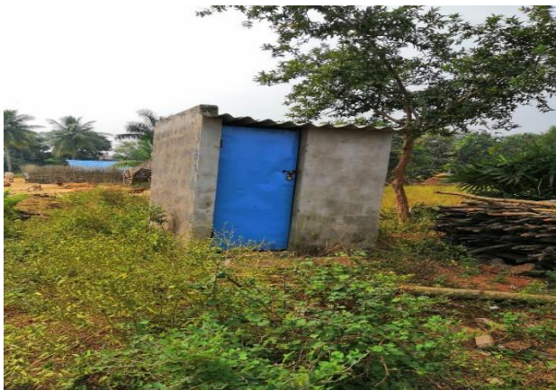
The ground reality of independent toilets built under the scheme Swachh Bharat
