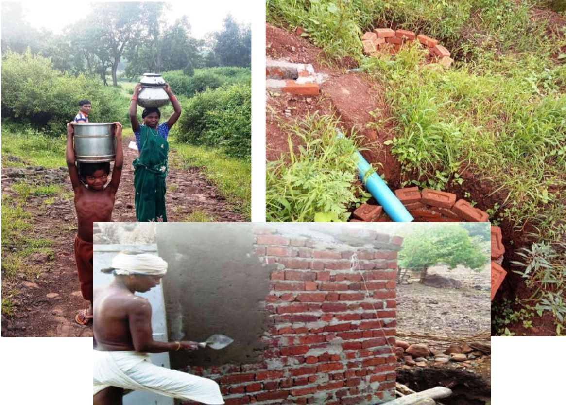
Picture 11: Construction of toilet by Baiga mason (under Souchalaya Nirman Yojana)
