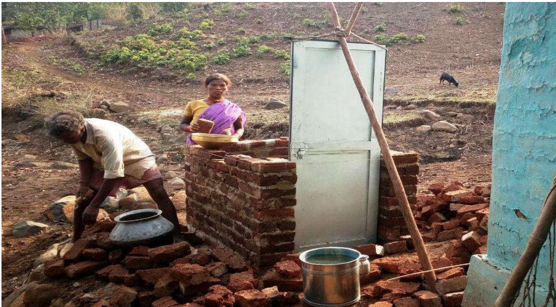
Picture 14: Construction of toilet under Souchalaya Nirman Yojana
