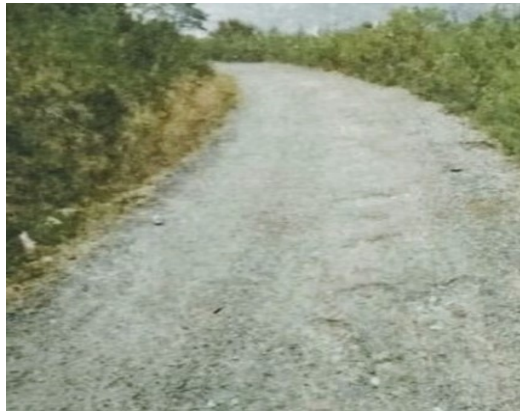
Roadway in Dhungsil
