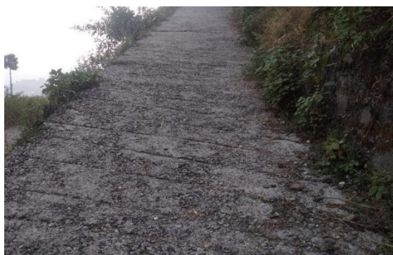
Roadway to Dhingsul village
