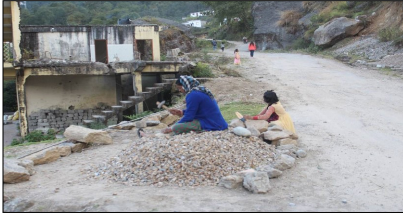
Women breaking the stone for Road Construction
