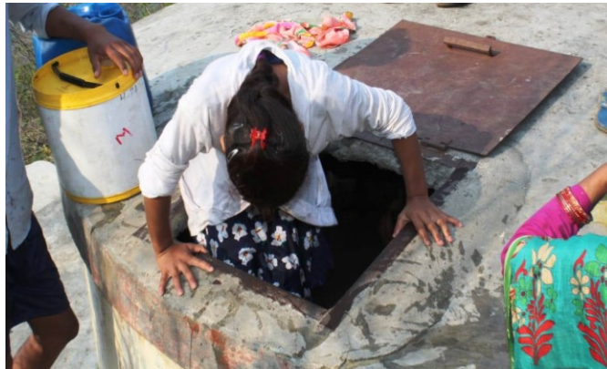
Emergency water storage units
