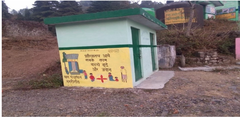
Toilets ( Primary School Malla Tirchakhet)
