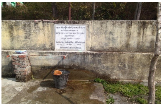
Water Storage Tank
