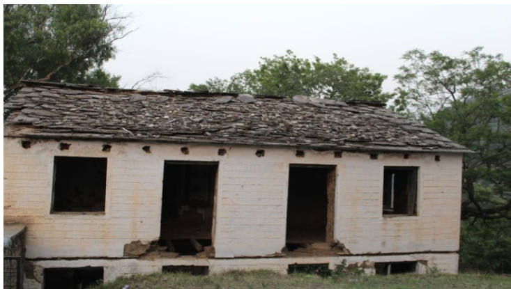
Abandoned house in Village Bitholi
