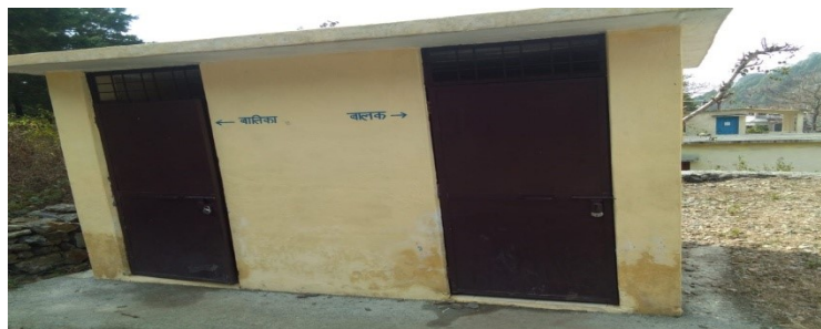
Toilets ( Junior High School Malla Tirchakhet)
