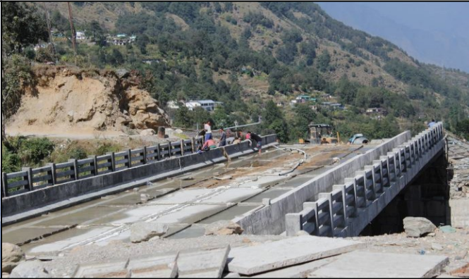
Construction of Bridge
