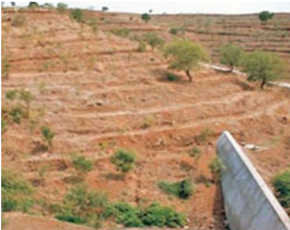
Figure 1-16 Contour Bunding 15
