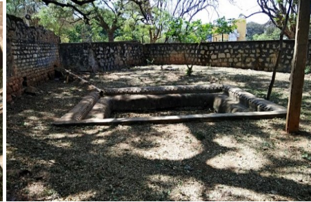
Rain Water Harvesting Pits
