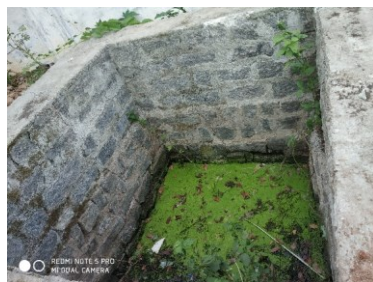
Rain Water Harvesting Pits
