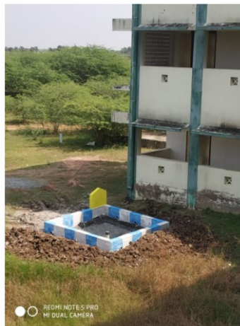
Picture 7: Rain Water Harvesting Unit was constructed after DSM visit at Govt. Arts College Thiruthuraipoonid, Tiruvarur
