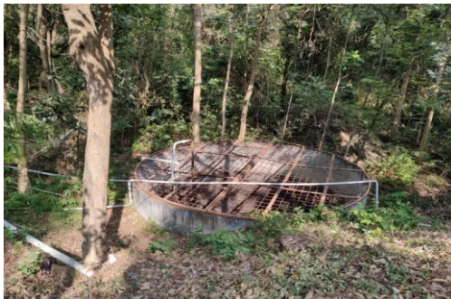
Rain Water Harvesting Pits
